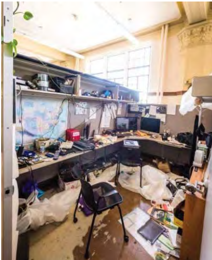
Office cubicles in the information technology area on the second floor were especially hard-hit with water damage.
