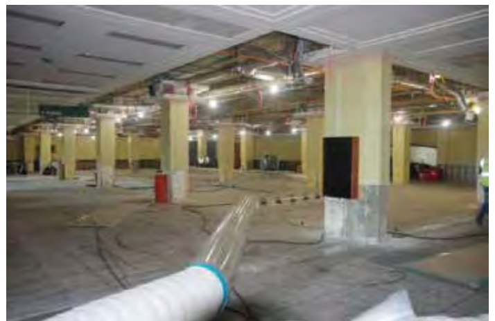
The second floor after the carpet, furniture, technology, drop ceiling system and some areas of drywall were removed.
