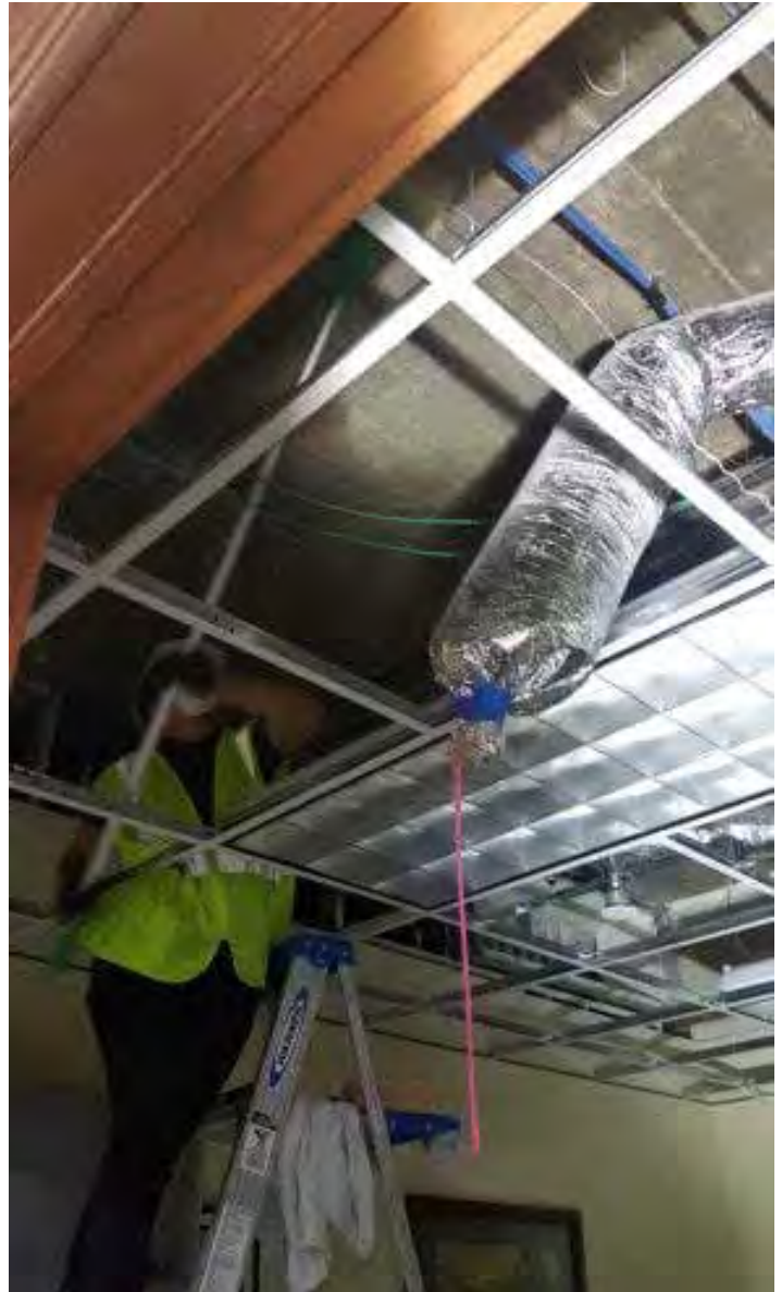
A crew member uses a chemical sponge to wipe down the ceiling and duct work.
