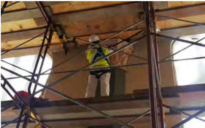
A worker removed paint from a plaster capital to allow water to evaporate from the walls more quickly.
