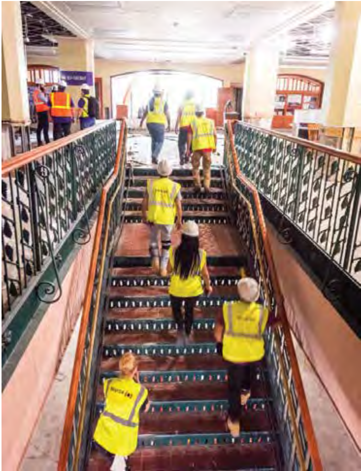
BELFOR workers make their way from the first floor to second.
