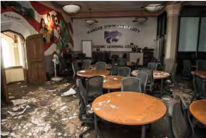
The Academic Learning Center was very near the site where the fire started on the roof and suffered extensive water damage.
