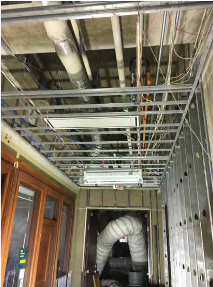
Second floor after ceiling tiles were removed.
